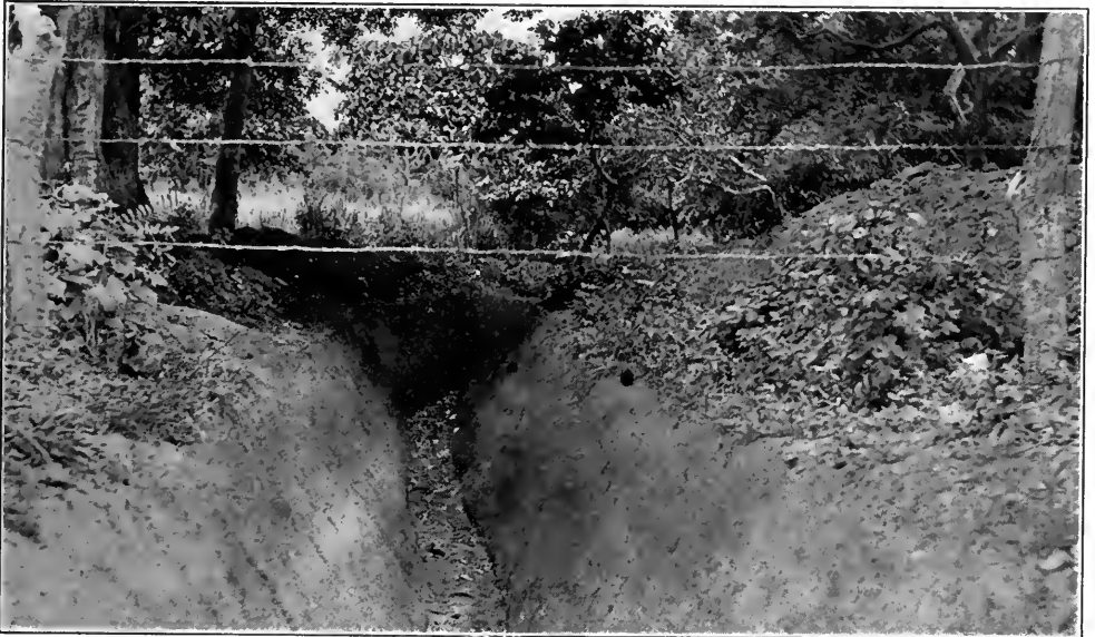
GOOD EXAMPLE OF "V" TYPE DITCH WITH SLOPE SLIGHTLY STEEPER THAN 45 DEGREES
